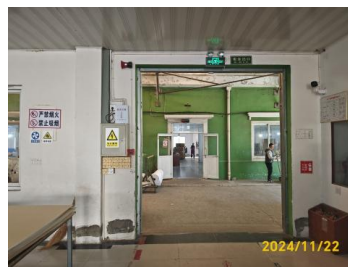
Emergency exit door.jpg
